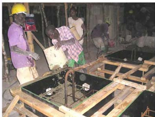
e) Making reinforced concrete anchors.
