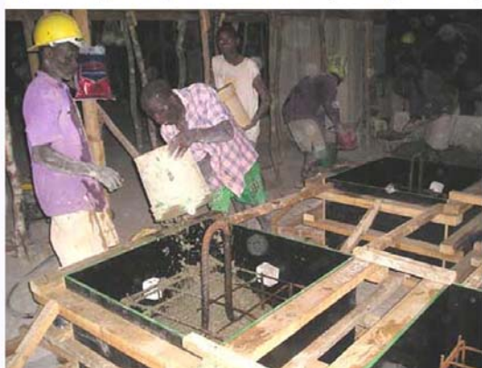
e) Making reinforced concrete anchors.
